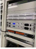
AEQ CROSSNET is a compact, 1RU intercom matrix with IP connectivity, based on Dante technology, compatible with the new AES 67 standard, carrying high quality audio suitable for broadcast. It also has high quality balanced analogue audio inputs and outputs and includes support for Kroma's legacy IP panels and interfaces with compressed
