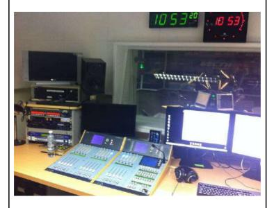
In 2014, the client acquired a redundant Intercom Conexia system for coordination between the studies and technical areas of the radio in Moscow. The installation has 51 user panels for TP4016 rack, one TP5024, 20 TP4216 desktop, and two linkers.
