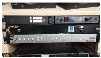
One Xpeak\_R rack terminal has been installed in the TV studio Production Control and another in the Radio Broadcast Control.
